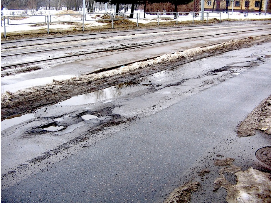
Fig. 3. First examined road segment with pothole
